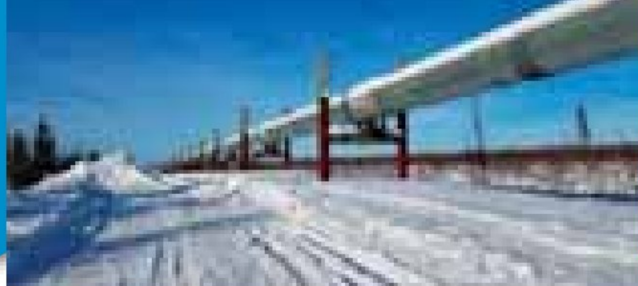
■ Figure 5.41 Trans-Alaska Pipeline
