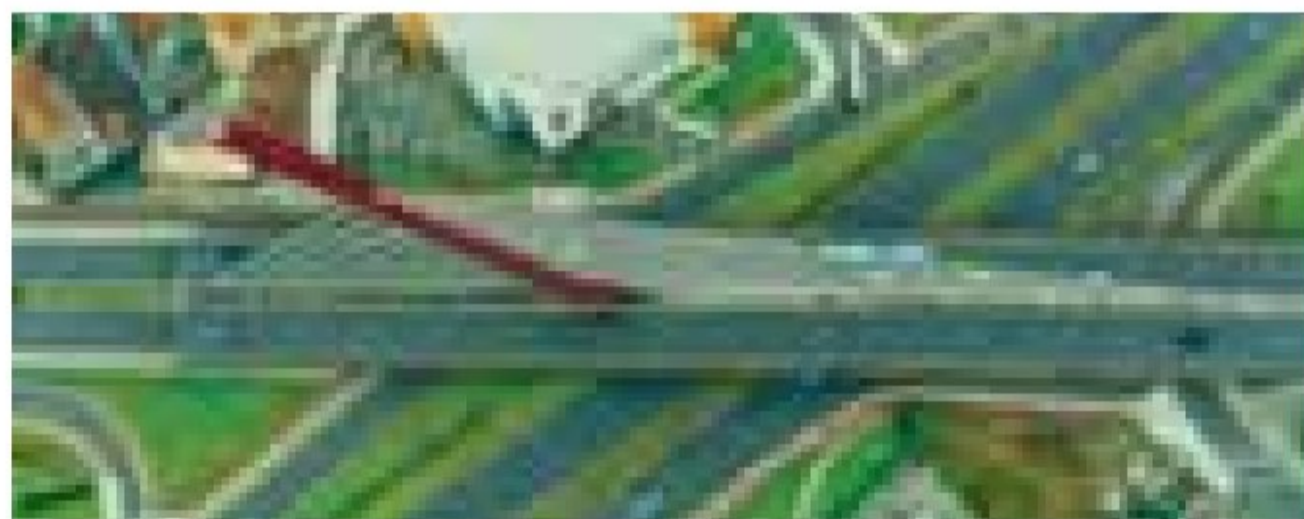
■ Figure 7.15 Aerial view of an avenue in Curitiba
